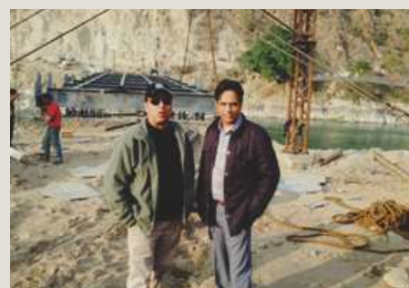
From Right: IECCD Chief Mr. Marasini and Under Secretary Mr. Pokharel in front of the bridge (under construction) at Khurkot of Sindhuli district
